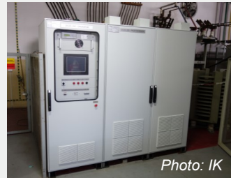
Fig 2. Energy storage DC/DC converter
