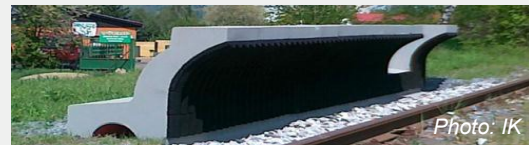
Fig 2. A low acoustic screen that protects the rolling noise emission
