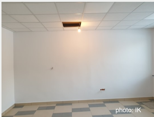
Photo 4. General view of a new laboratory room in Building 26
