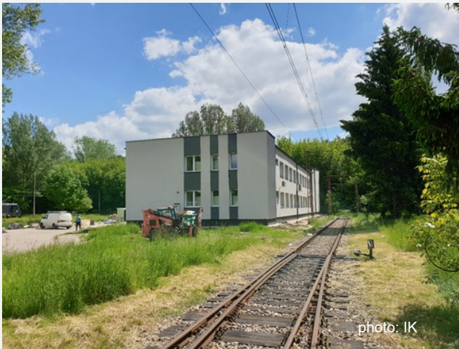
Photo 1. General view of the modernized building 26 of the ETO
