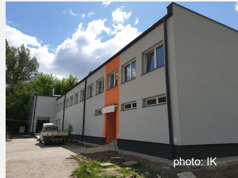
Photo 2. General view of the modernized building 26
